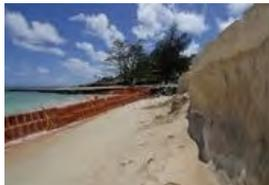
The "sand grabber" extending from Kailua Beach's small boat launch ramp was installed 30 years ago to stave off erosion and has been covered by sand for so long that most beachgoers forgot it was there. Now, the sea has reached beyond the grabber's concrete blocks and eaten away the beach, leaving a 5-foot dropoff.
